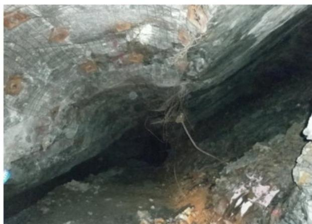
ABOVE: A mined area from Citigold's test mining showing the floor of the level drive, and the stope voids (ore extracted area) above and below the level. The ore has been cleanly extracted, showing how the mining method minimizes dilution by maintaining a narrow stoping 'slot' width.
