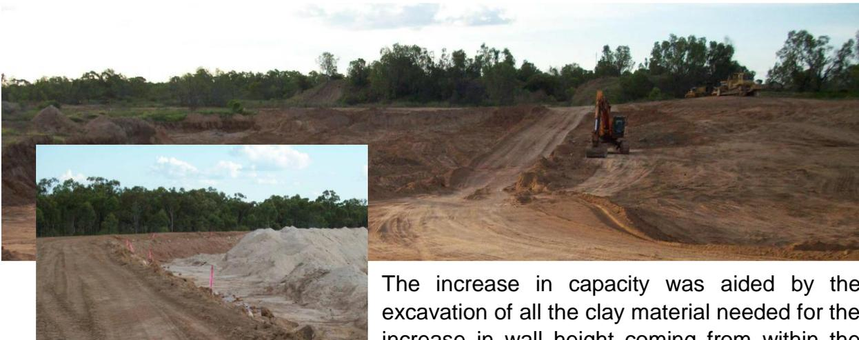
The increase in capacity was aided by the excavation of all the clay material needed for the increase in wall height coming from within the perimeter of the northern end of the TSF. This efficiency created additional internal volume with overall capacity increased to almost 400 mega litres.
